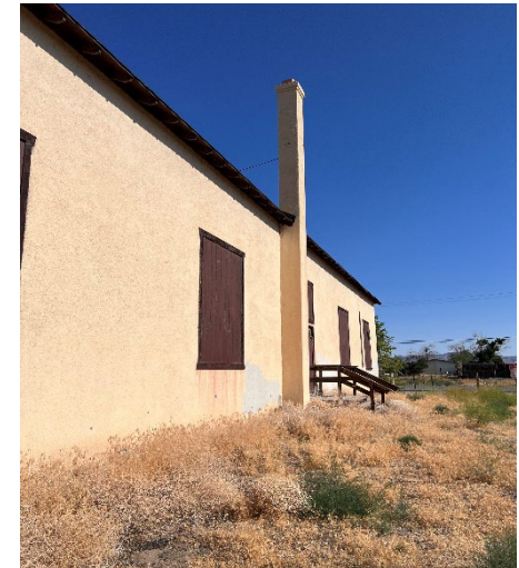
East facing side of building on the Subject Property
