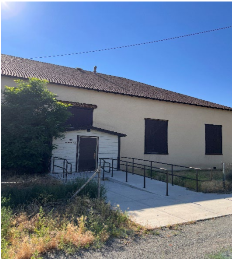
West facing side of building on the Subject Property
