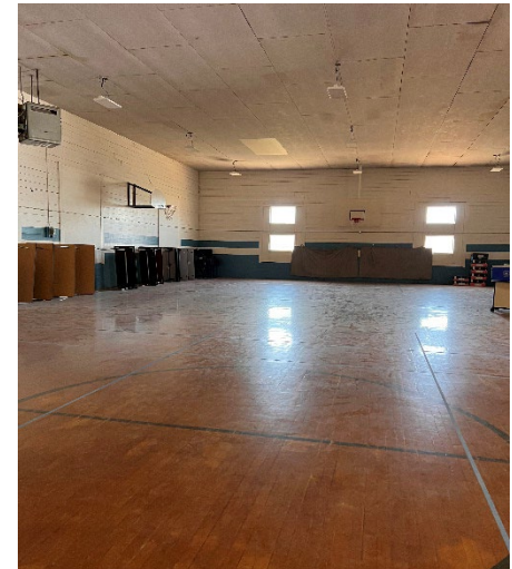
Gymnasium facing south
