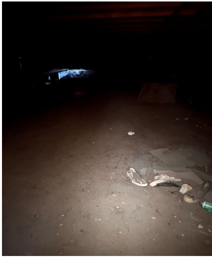
Crawl space area on the Subject Property
