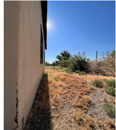
South facing side of building
