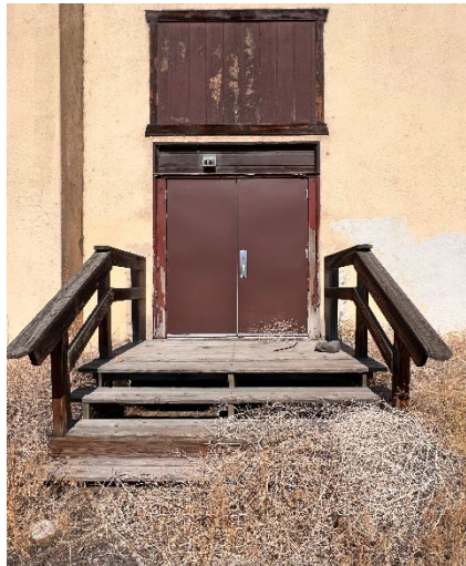
Back (eastern side) door on the Subject Property
