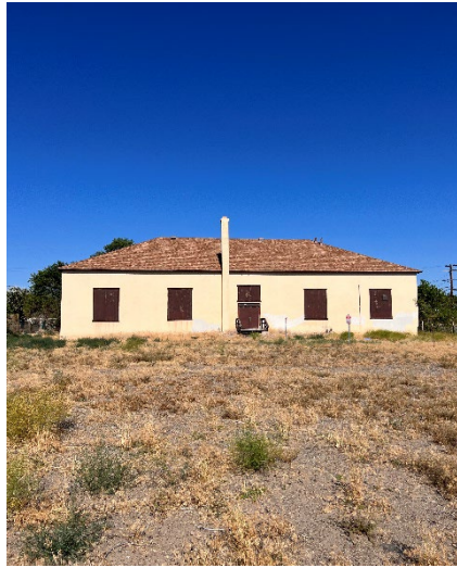
Eastern facing side of the Subject Property (facing west)
