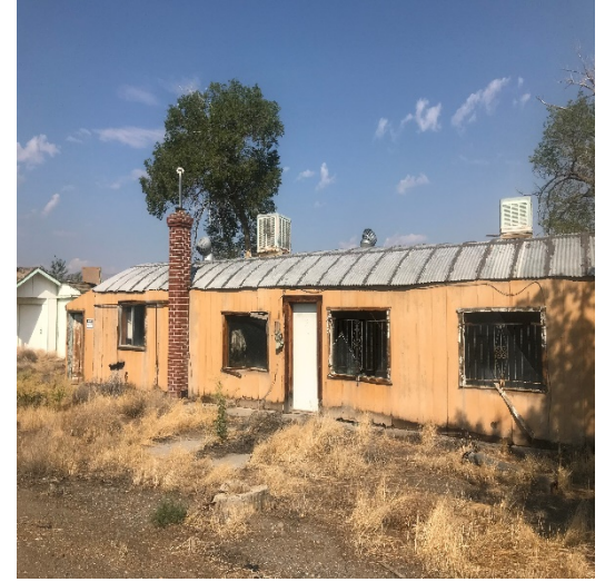
Building on the Property
