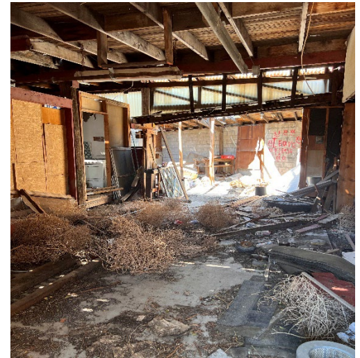
Interior of building on Property
