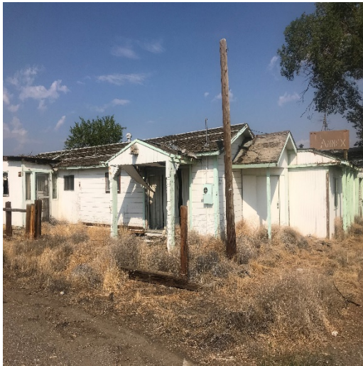
Building on the Property
