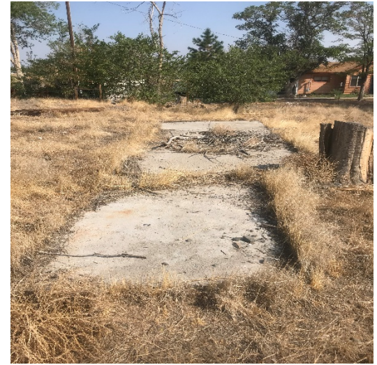
Concrete pad of former building structure located eastern portion of the Property
