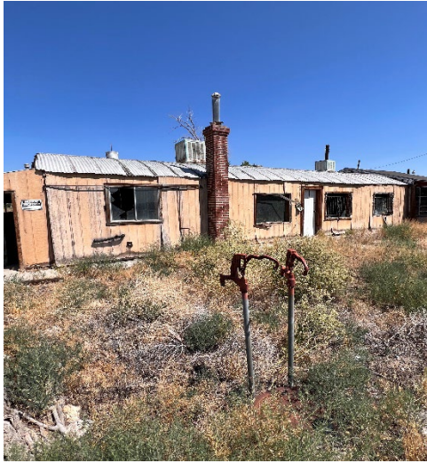
Building structure on the Subject Property
