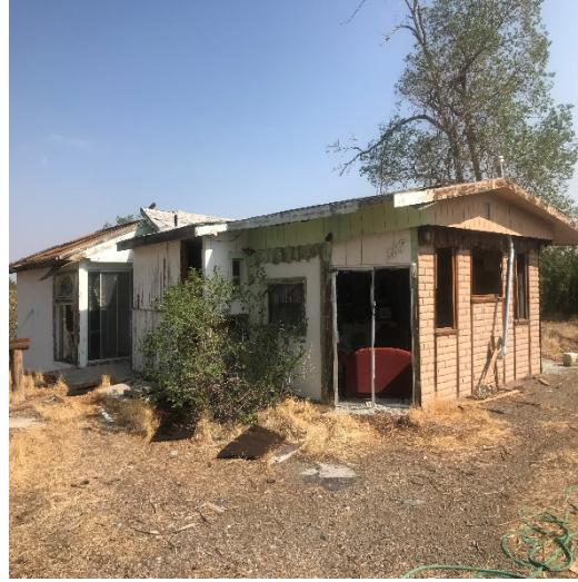
Building on the Property
