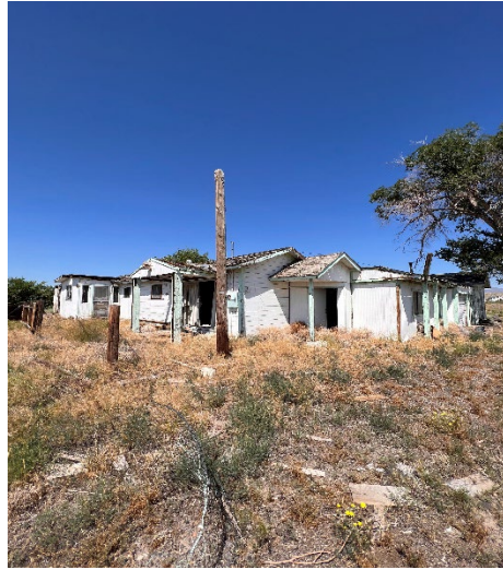
Building on the Property
