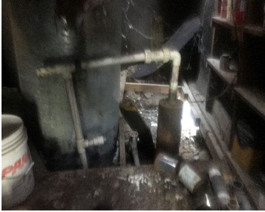
Domestic well on the Property
