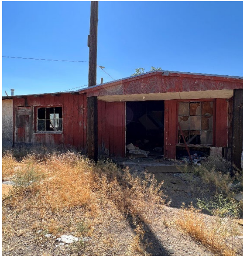
Building on the Property
