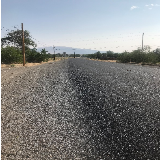
Main St. facing east
