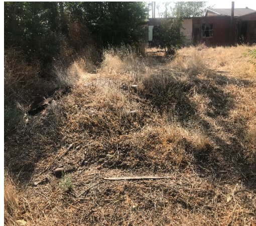
Dirt mound on the Property. Potential buried tank and/or fill material
