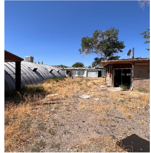
Buildings on the Property facing west
