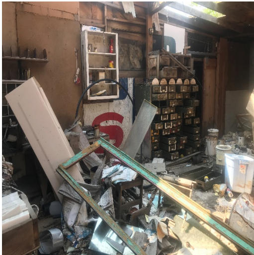
Interior of building on the Property
