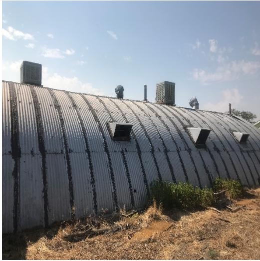
Building structure on the Property
