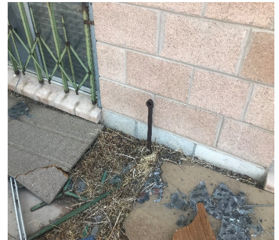
Potential heating oil tank vent northwestern portion of the Property
