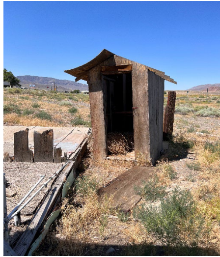
Outhouse structure on western portion of the Property
