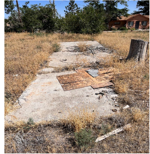
Concrete pad of former building structure located eastern portion of the Subject Property
