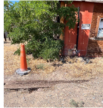
Potential buried tank area on the Property
