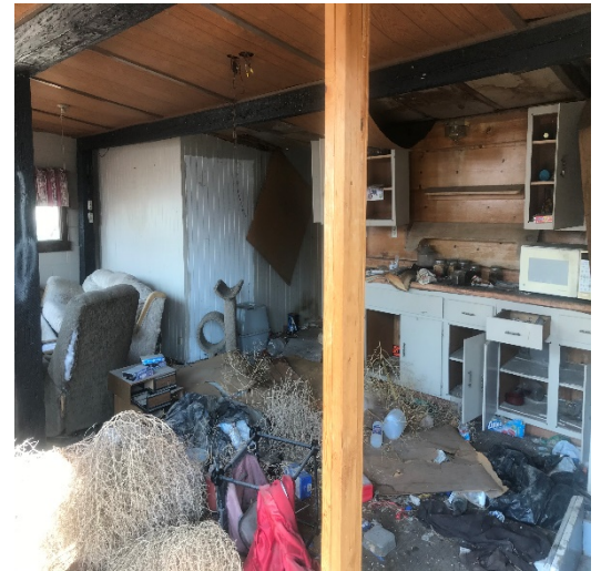
Interior of building on Property
