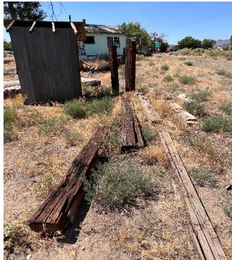
Discarded railroad ties on the Property
