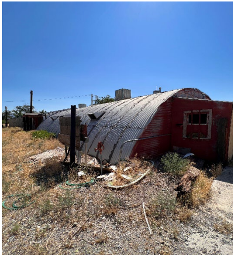
Building on the Property
