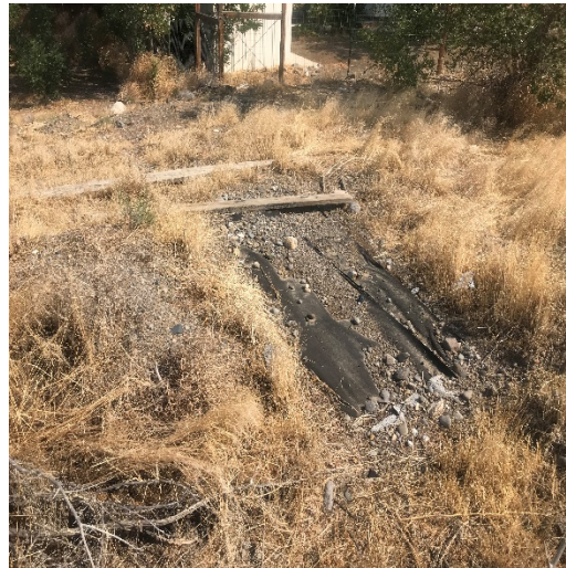
Potential buried septic tank area located northeastern portion of Property
