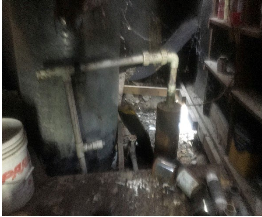
Domestic well on the Property
